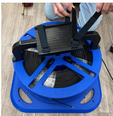
Step 8: Secure the HyperDROP™ MST, HyperDROP™ Squid, or other end of the drop cable to the tray with provided Velcro® straps.
