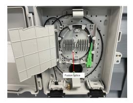
5. Attach the incoming cable to the tie wrap area (remove tray to place zip ties):
