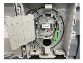
**Splice incoming to outgoing:** Push the splice sleeves into the splice chip holder above the slack tray. Run excess incoming fiber clockwise and outgoing counterclockwise around the round slack tray in the middle
