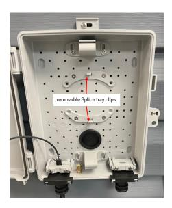
**Pigtail installation:** Push the splice sleeves into the splice chip located just above the slack tray at the top of box. Plug the connector into the adapter. Run excess fiber clockwise around the round slack tray.
