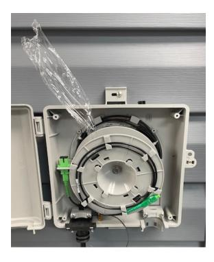
8. Punch hole through the right grommet or us bug grommet and guide outgoing fiber through the entry.
