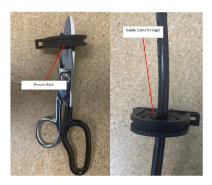
(B) when using bug grommet slide cable through grommet before pushing in place secure with zip tie.
