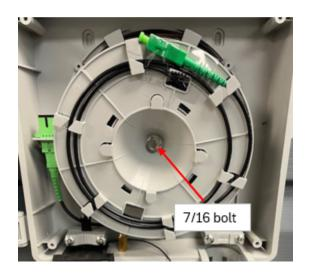
11. Close, tighten, and secure the outside cover using the security bolt.
